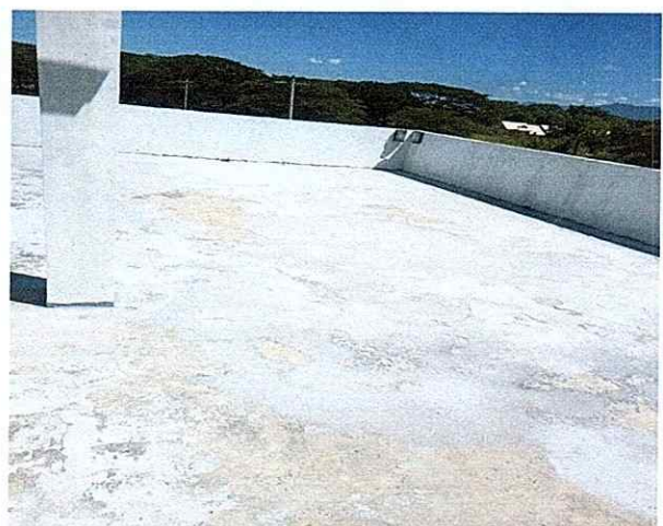
Fig. 2 Major leak from the roof deck especially during heavy rain.
