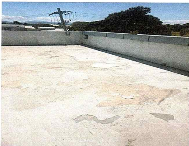
Fig. 2 Major leak from the roof deck especially during heavy rain.
